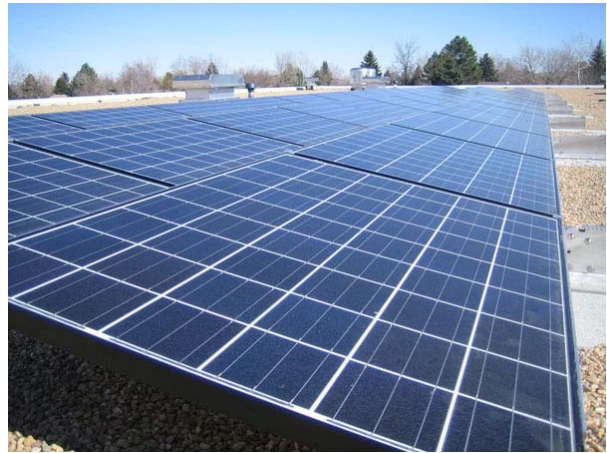
A 9.8 kilowatt photovoltaic system was installed on the roof of the new wing
