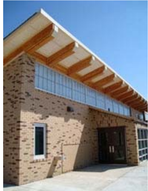
The classroom addition at Lafayette Elementary features ample
