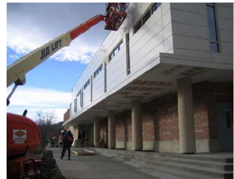
Sandstone used for the veneer, was recycled from the exciting building
